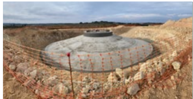
Image 2.1 Concreting the SO2 wind turbine (Solans wind farm).
